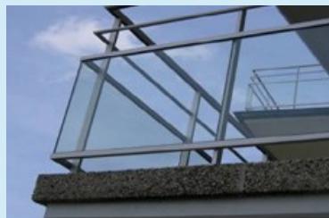
Figure B107 — Glass balconies should be 50% tinted
