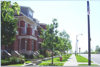
Figure B85 — Hurontario Street South East side
