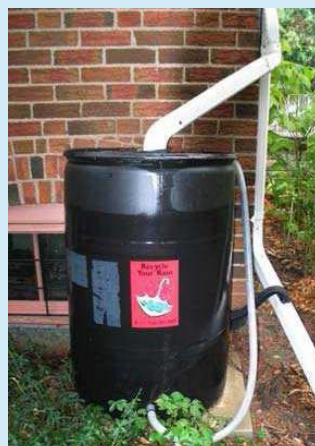
Figure D3 — Typical rain water barrel
