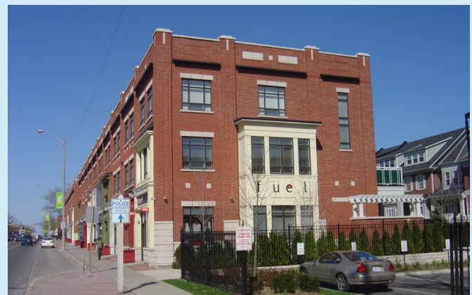
Figure B34 — Image of the existing mainstreet building
