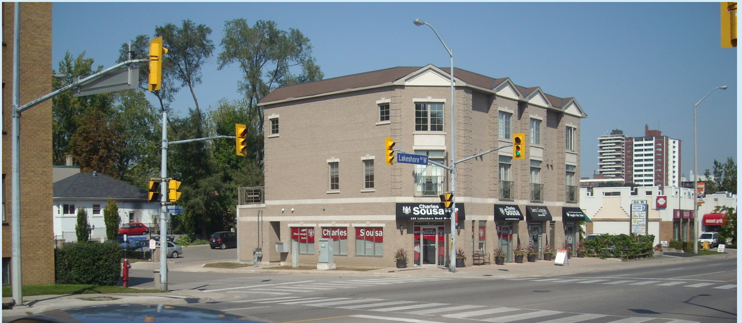
Figure B16 — Mainstreet Precinct, Mississauga Road and Lakeshore Road West. New construction.
